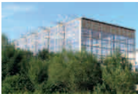
Herzog + Partner: Training center for the Bavarian mountain rescue, Germany (2006/08)
